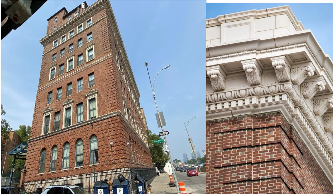
Former Gouverneur Dispensary. 7 Gouverneur Slip East and detail. Opened in 1914 with 3 stories; later enlarged. Now houses Lower East Side Center – Su Casa. (Photos: D.Wye and Boston Valley Terra Cotta)
