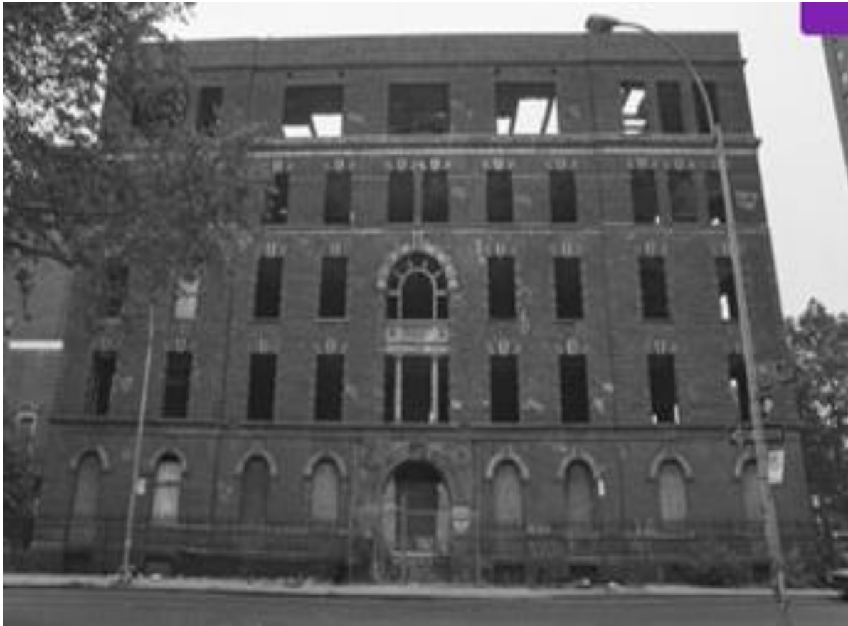
Gouverneur Hospital, abandoned from 1981-1992. (Photo: Larry Racioppo, HPD)
