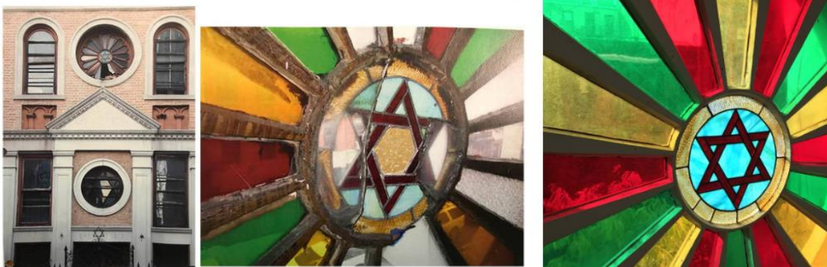
Façade and close-up of top rose window before 2012 restoration and after. (Photo-Stanton Street Shul website)
