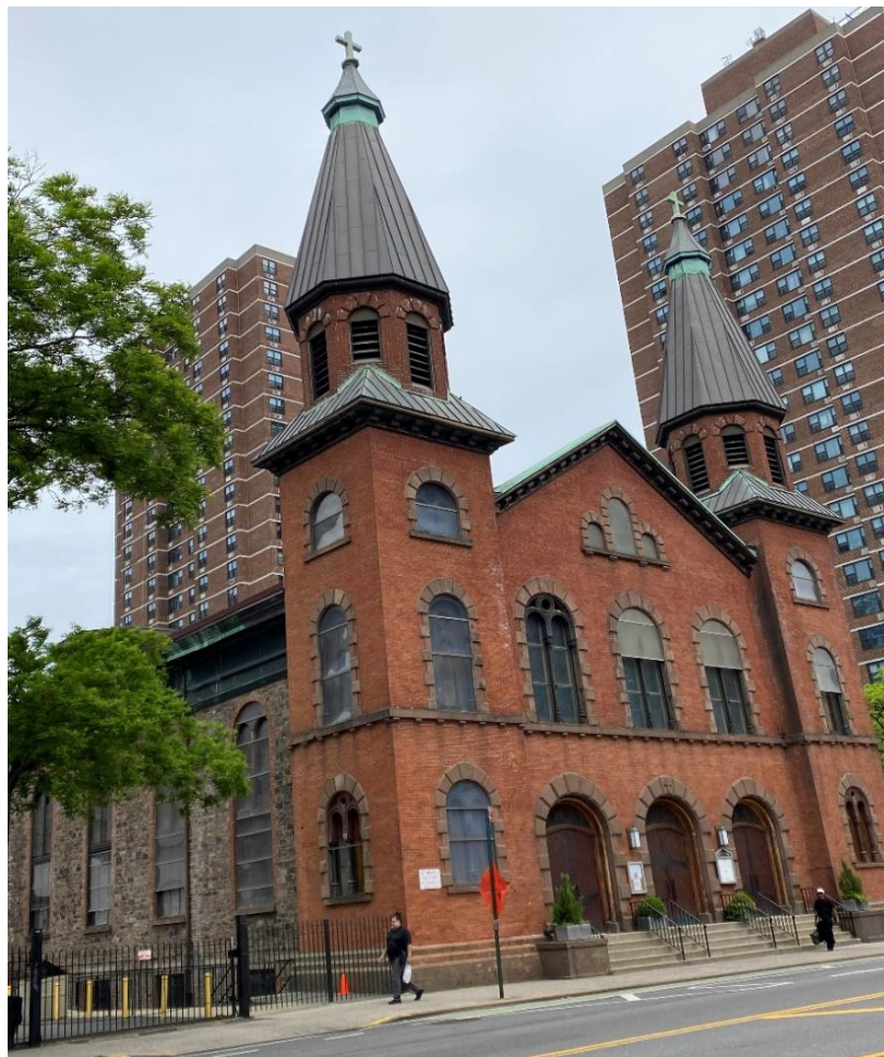
Church of Saint Mary, 438-440 Grand Street. Fieldstone walls from 1833; brick and brownstone facade from 1864. (Photo: D.Wye)
