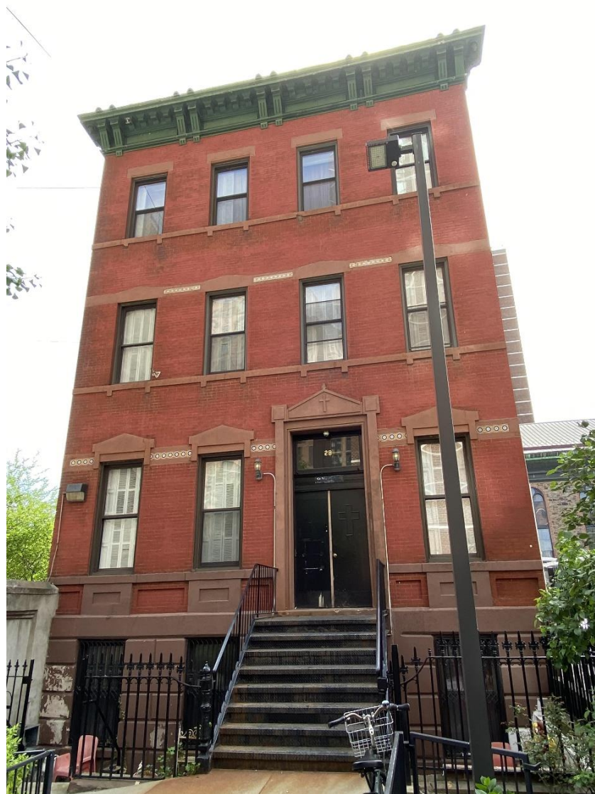
Rectory on St. Mary's campus. Former 1850 row house at 28 Attorney Street, purchased by St. Mary's for a rectory in 1865. (Photo: D. Wye)
