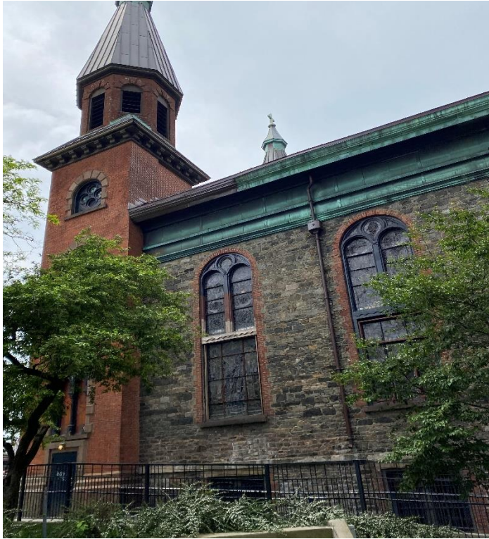
St. Mary's, view of east side. (Photo: D. Wye)
