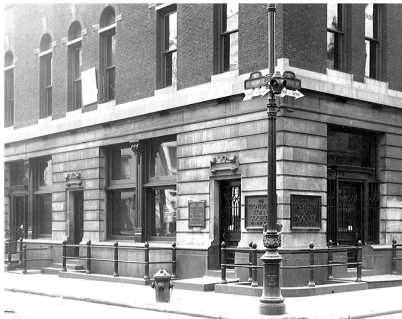
First office of The Provident Loan Society in rented quarters at the University Settlement on the Lower East Side. Signs for the Society are on both sides of the building's corner. (Photo: Provident Loan Society website)
