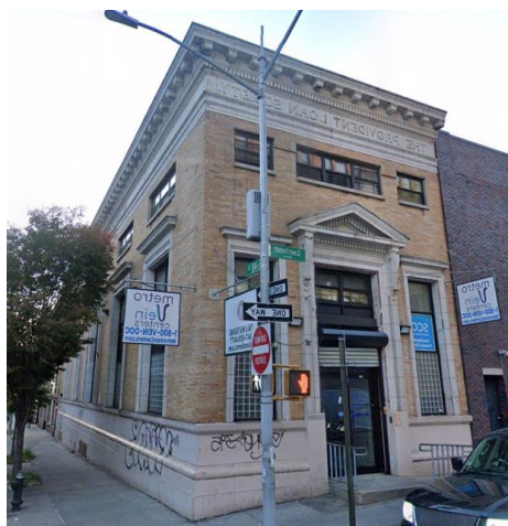
Former Provident Loan Society building at Courtlandt Avenue and 148th Street (Photo: Google Maps)
