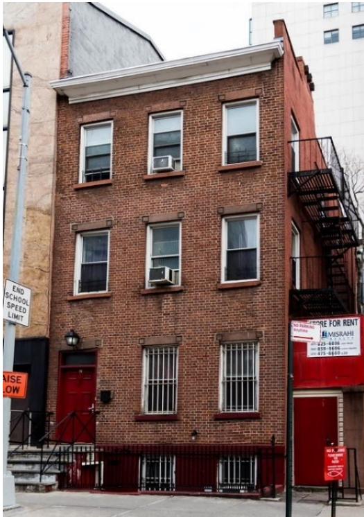
No. 2 Oliver Street. 1821. Building raised in 1850. Builder: Robert Dodge. (Federal/Greek Revival). Photo: Bruce Monroe
