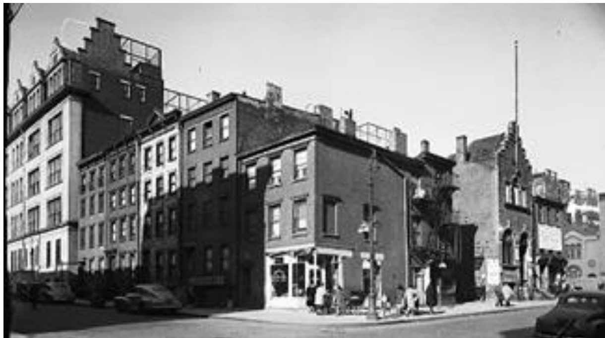
SE corner, Oliver and Madison Sts. 1948. Demolished 1950. 28 Oliver-2nd building after P.S. 1 (left). Downtown Tammany Club (stepped, gable-front roof)-3rd building on Madison St. (right). Photo: Pratt: LaGuardia-Wagner Archive
