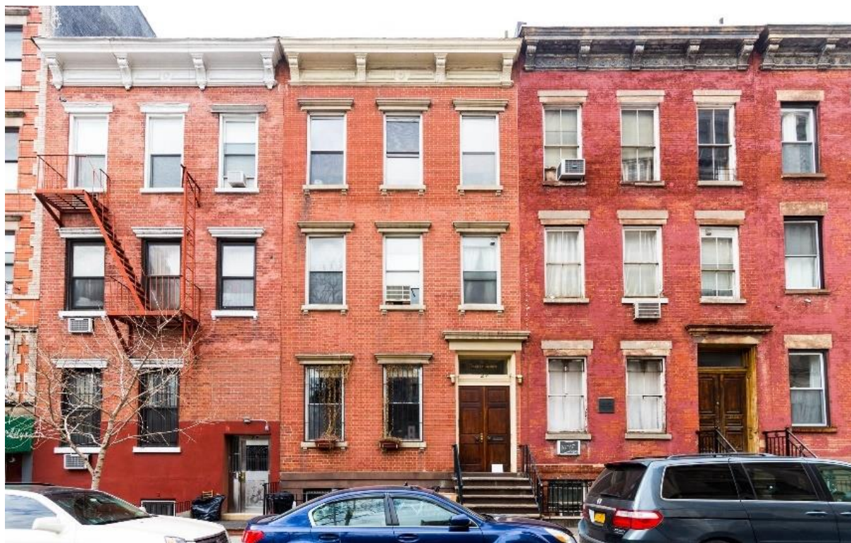
From left: Nos. 29, 27, 25 (Smith residence) Oliver Street. (Partial view of nine brick row houses). Photo: Bruce Monroe
