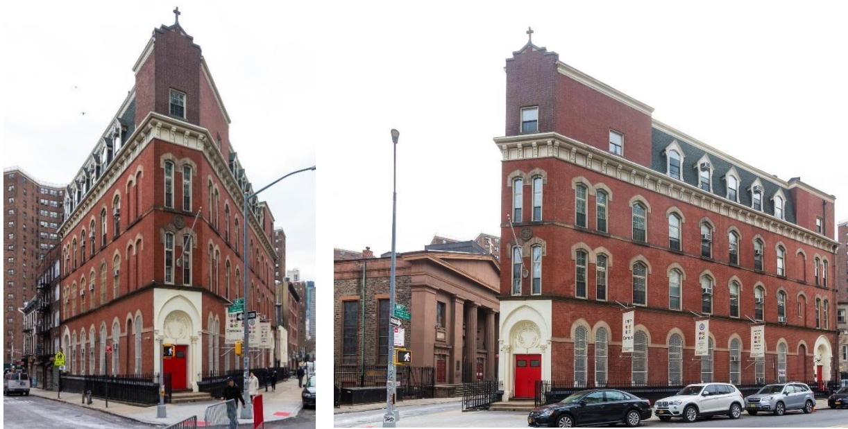
Former St. James School (now Transfiguration School). 1868. Corner of James Street and St. James Place. (Eclectic). Photos: Bruce Monroe
