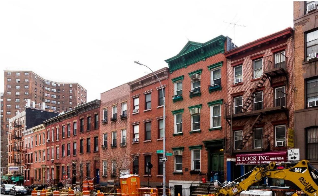
Left to Right: Nos. 29-13 Oliver Street. Early 19th c. Buildings raised c. 1860s-1880s. Photo: Bruce Monroe
