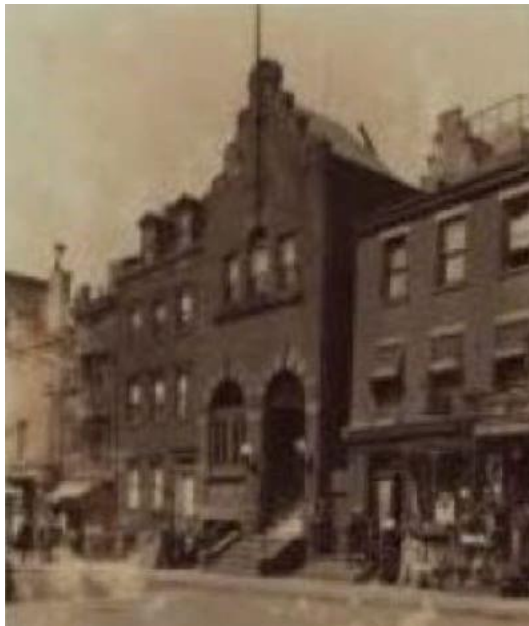
Downtown Tammany Hall Clubhouse. 59 Madison St. Demolished 1950 for current playground. Photo: NYPL
